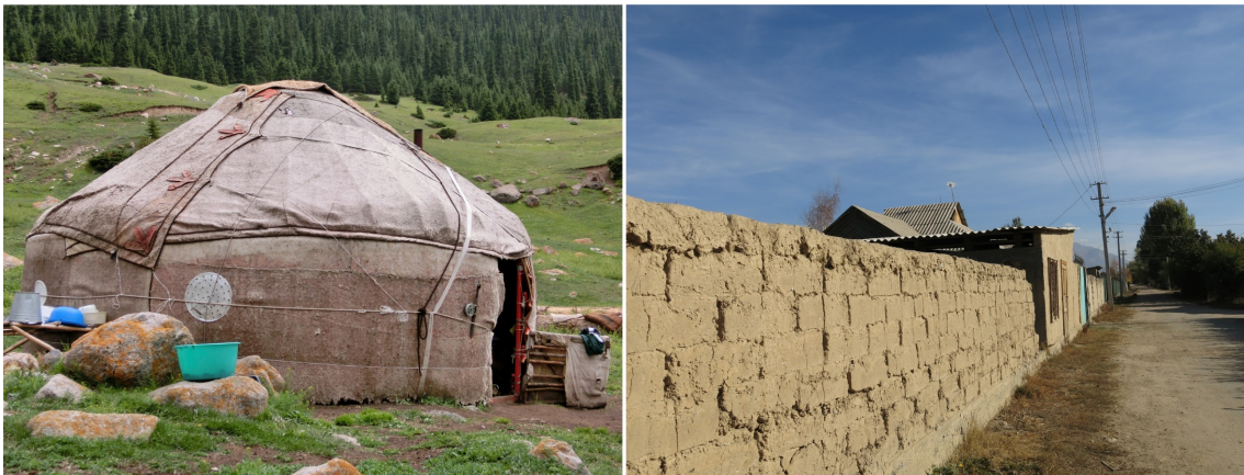
Figure 3.3: Traditional building techniques. To the left: a yurt. To the right: a wall made of clay and straw, like some buildings which are still built in the countryside.
