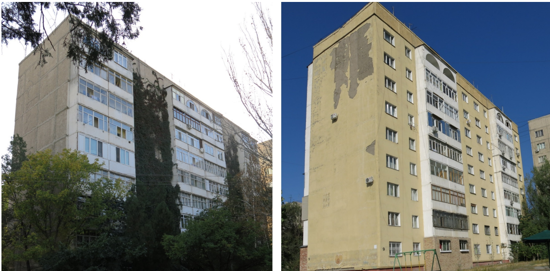
Figure 7.1: The examined buildings. To the left: House 2. To the right: House 9.
