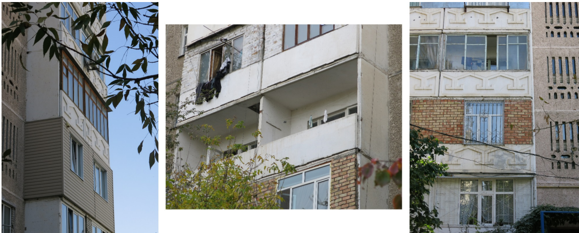
Figure 8.11: Different modification of balconies from Asanbay microregion. The balcony in the middle, without windows, got the original shape of a balcony on building type 105. This is however now seen on only 6 balconies on both houses.
