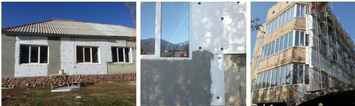
Figure 3.4: Examples of insulation improvement. Pictures to the left and in the middle: retrofitting of a building on the countryside by adding insulation. To the right: a brick-building being constructed in Bishkek.
