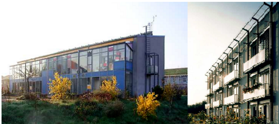
Figure 3.13: The Passive house, Kranichstein (Feist 2006b)
