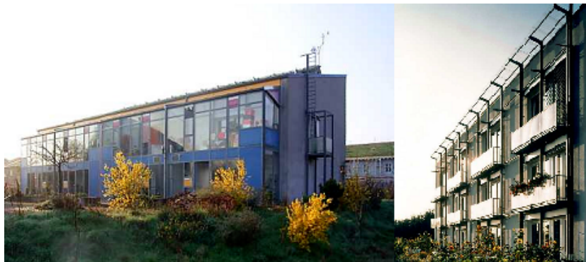
Figure 2.3: Passive house in Kranichstein - North side and southern facade (Feist 2006b)
